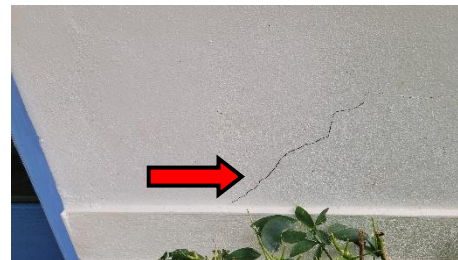
Settling Crack
