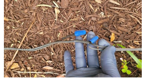
Damaged/Split line.
