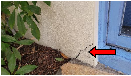
Settling Cracks
